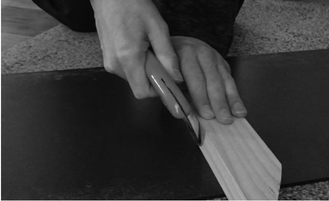
Fig. 2. Cutting fibre cement slate using a scriber
