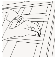
Nailing verge units
