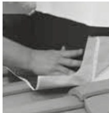
Form the material and cut to shape required
